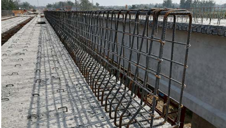
astm a615 rebar bridge construction
